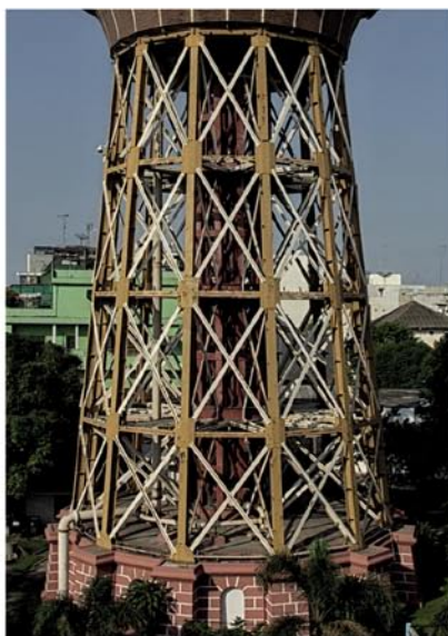
The sturdy construction of this tower's poles can support a large tub with 1200m 3 of capacity.
