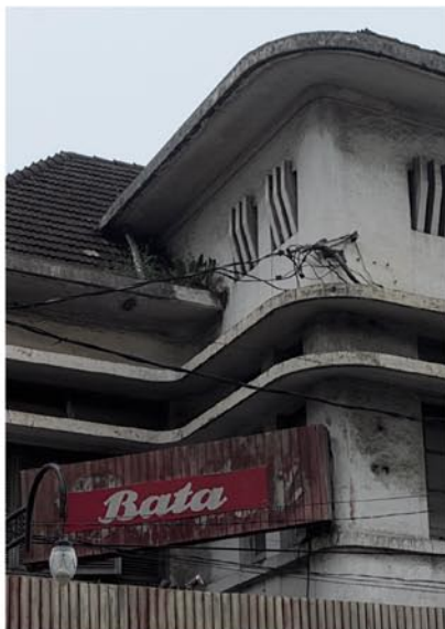
The top of the building which also serve as ventilation and air circulation.
